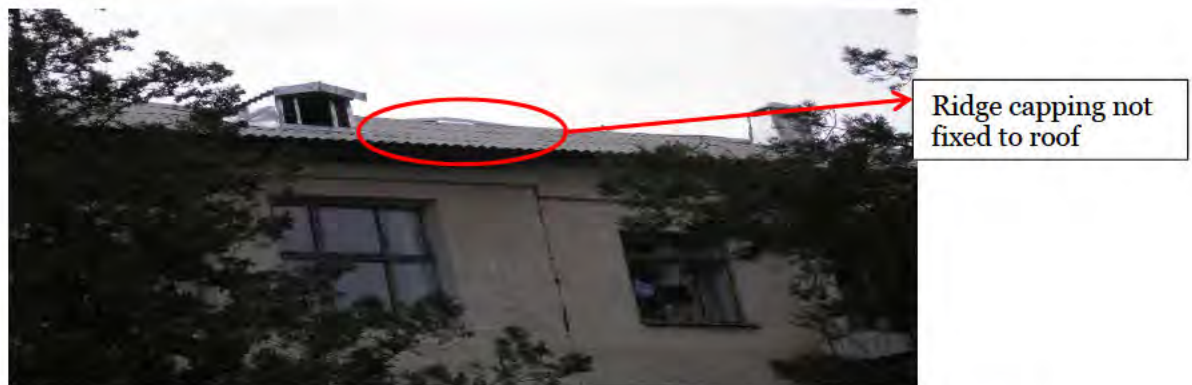
Fig. 30 - Poor quality roof renovation
